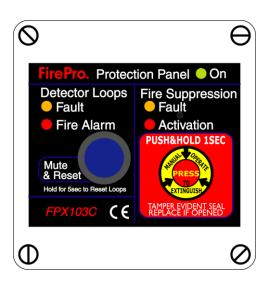
Shutdown and delayed firex activation improves effectiveness and saves cost of extra extinguishant. Most existing extinguishing systems release the agent into a high airflow environment which makes it almost completely ineffective. Given that a 7 Liter 4 stroke engine at 3000RPM (that's 50revs/sec) aspirates 175 Liters or 0.175m<sup>3</sup> of air *per second*, add to this ventilation fan flow and the necessity for a shutdown with engine/fan spindown delay before activation is obvious.
